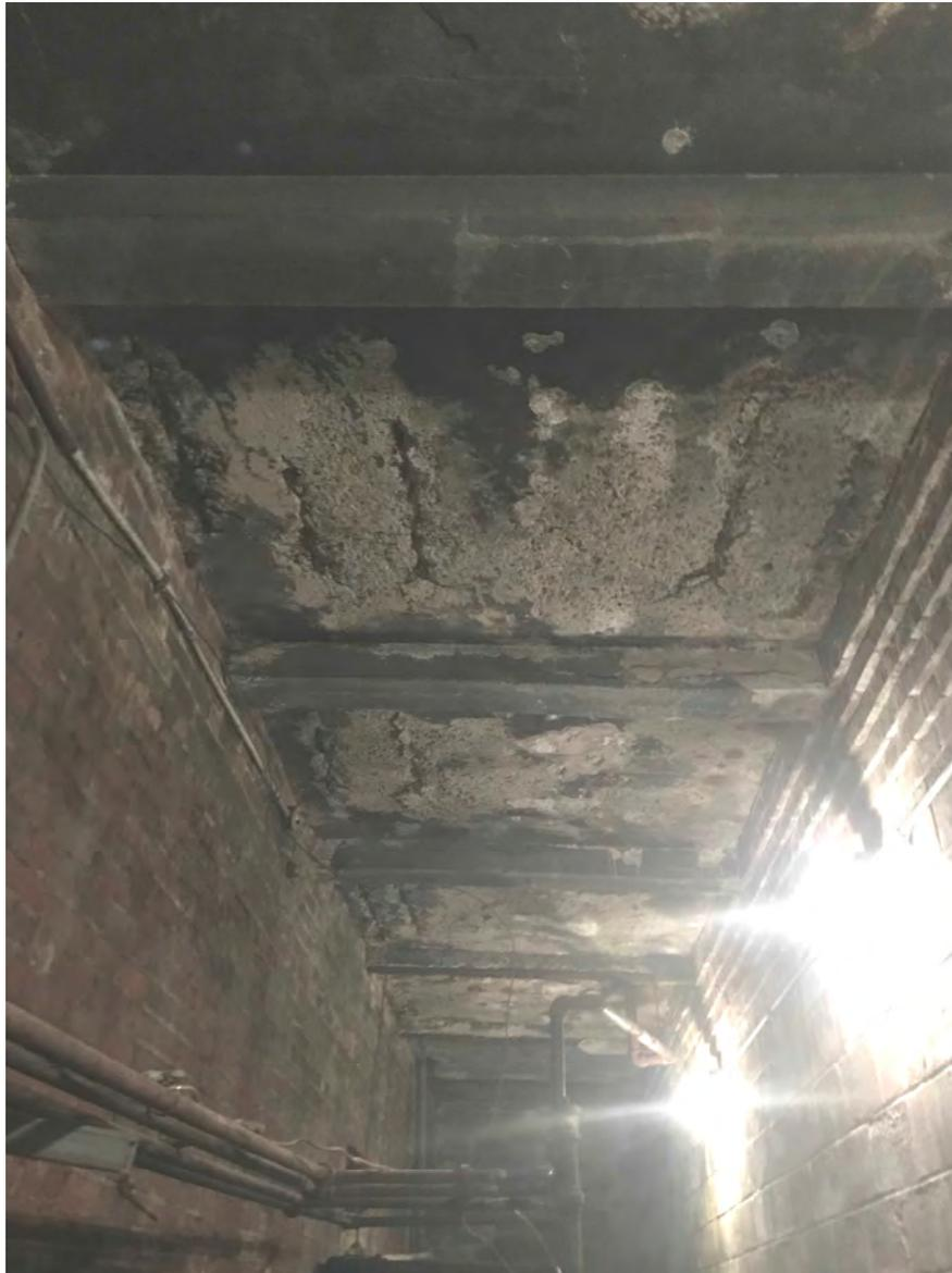
This is a photo of the ceiling of the vault looking west. The ceiling shows some of the steel beams. The first two are still covered with cement, the third one has lost its cement.
